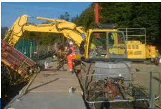
■ Installing SBMA anchors on the Crag End landslide in Northumberland
