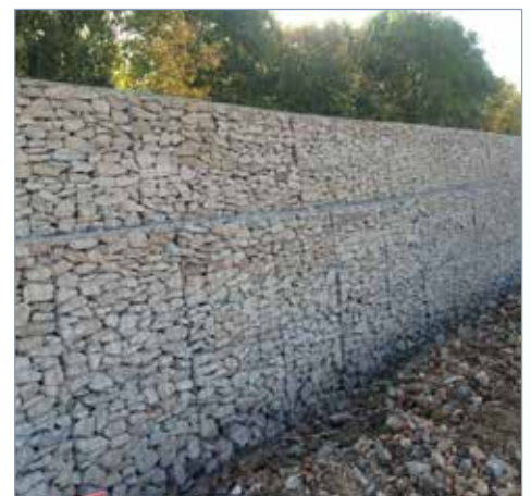
■ Gabions are a popular choice for highways projects
