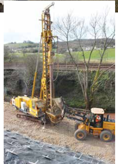
■ Installing vibro stone columns on the Kingskerswell bypass in Devon
